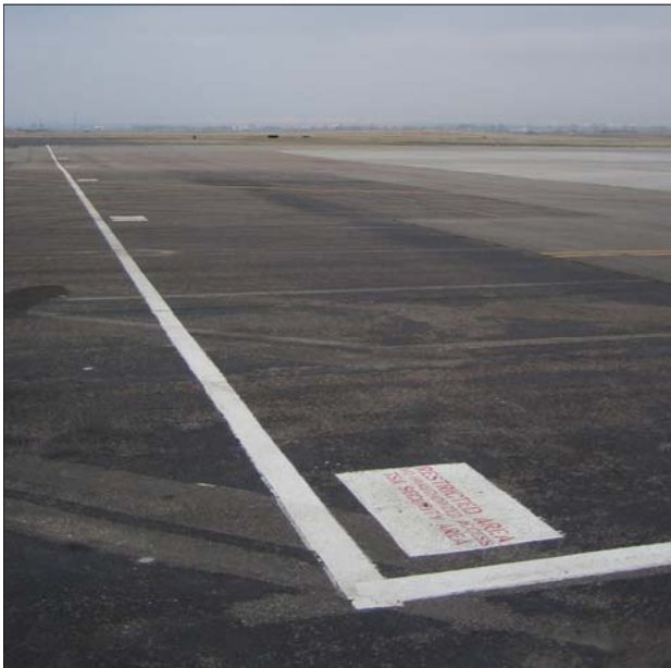
Another view of TSA Security Area lines. No unauthorized access from any side when any commercial carrier is on the ground.
