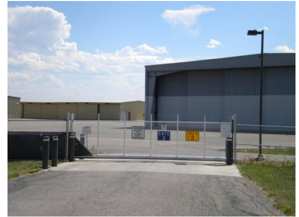
Gate #3 Fire Station
