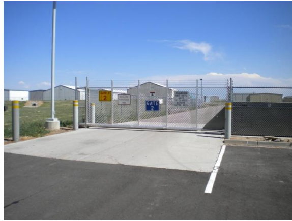
Gate #2 FBO Parking Lot
